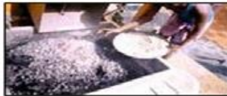
Shredded polymer waste is added to heated stone aggregate for 30-40 sec and mixed for uniform coating
